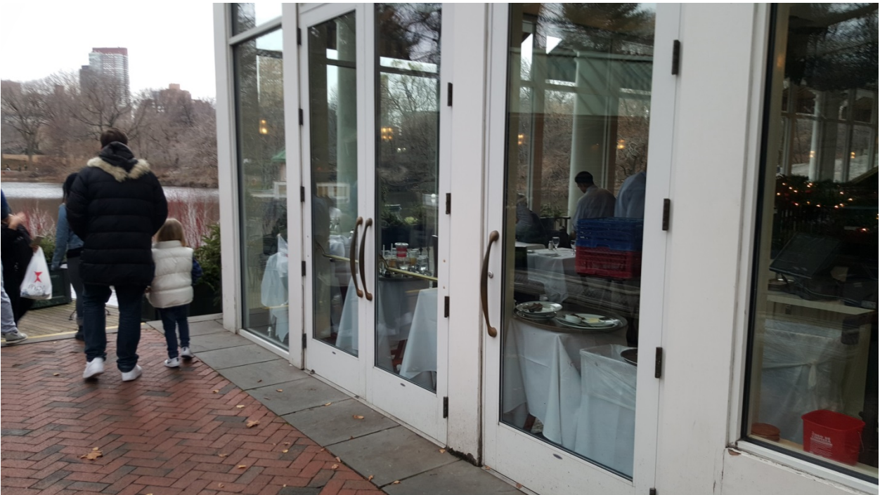
Figure 3 - Photograph of Patio Doors from Brick Patio; visible are the equipment blocking access to the doors. Taken Dec. 26, 2015.
