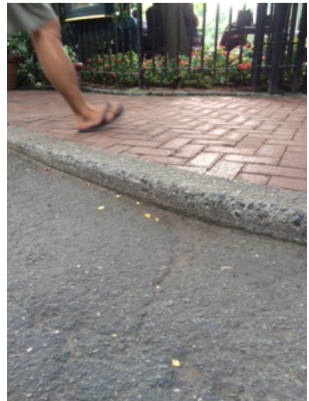
Figure 1 - Photograph of Curb Outside Restaurant; visible is the step up from the street to the brick entrance level and poured asphalt ramp. Taken August 27, 2015.
