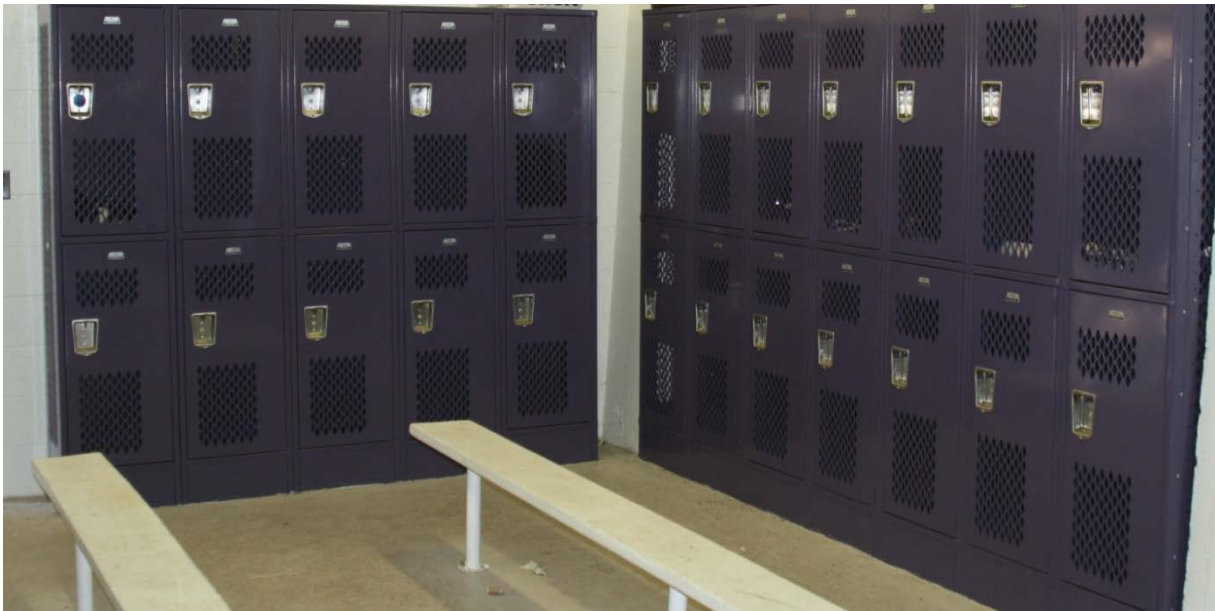
Locker room, Cardozo Senior High School, 1200 Clifton St. NW Washington, DC, Ward 1
