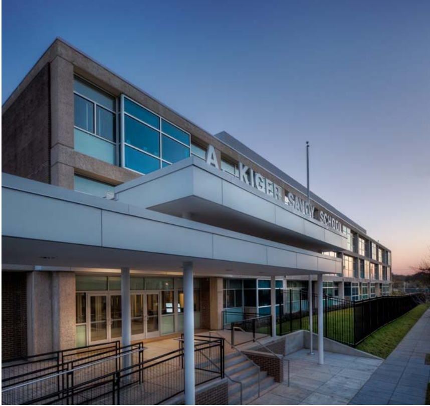
Entrance, Savoy Elementary School, 2400 Shannon Pl. SE, Washington, DC, Ward 8
